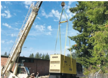
Central Kitchen: New generator installed
