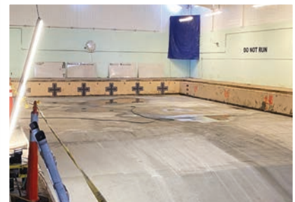
View following demolition of the old pool floor and installation of the new concrete pool floor.
