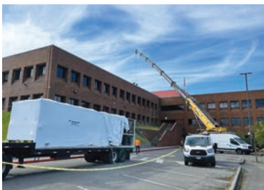
South Kitsap High School: HVAC Chiller replaced
